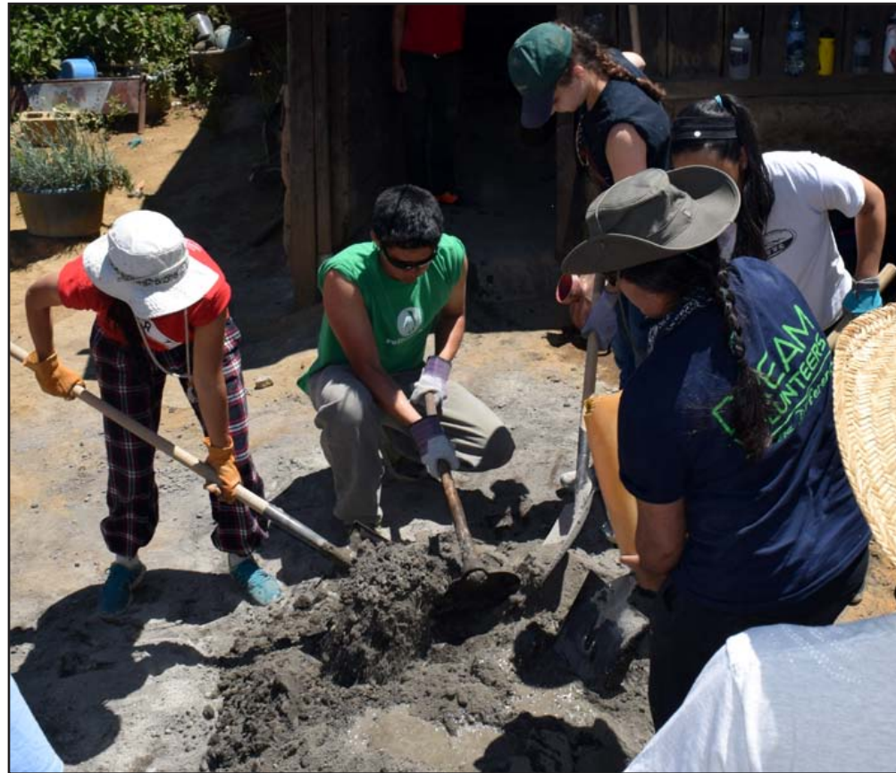
Cory Gong (green shirt) and his fellow Gunn High students mix cement on the ground for the foundation, using just shovels and their bare hands.
